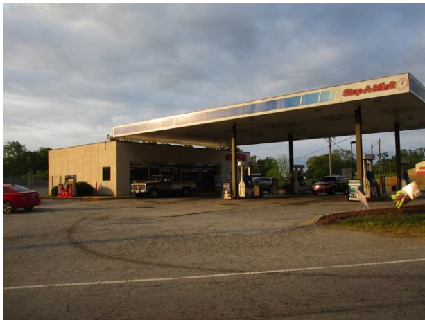
Typical commercial/retail uses in Subject's neighborhood
