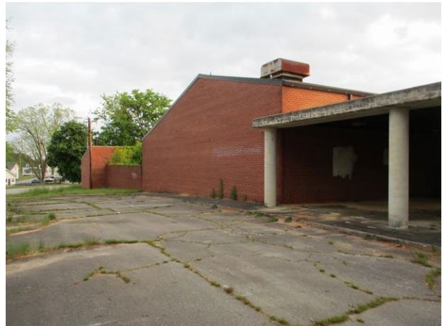
View of existing improvements on Subject site
