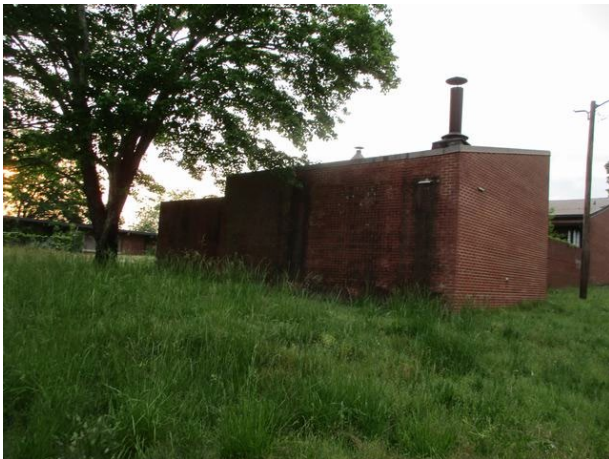
View of existing improvements on Subject site
