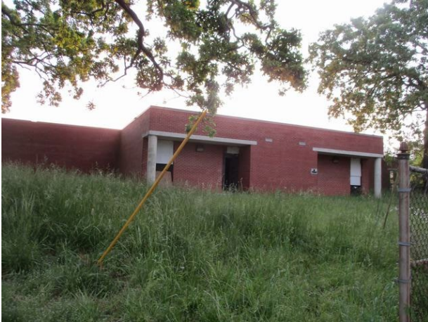
View of existing improvements on Subject site
