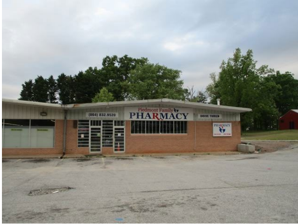
Typical commercial/retail uses in Subject's neighborhood
