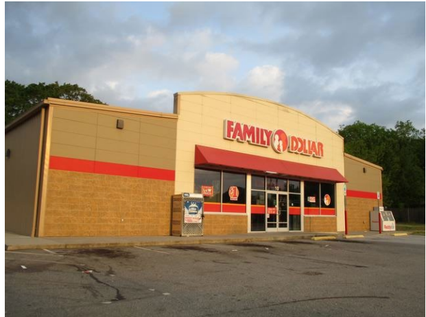
Typical commercial/retail uses in Subject's neighborhood
