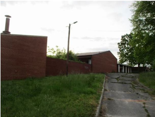
View of existing improvements on Subject site
