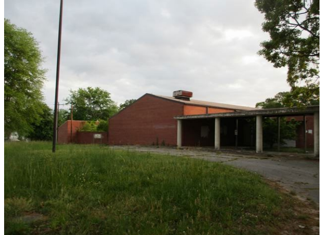
View of existing improvements on Subject site
