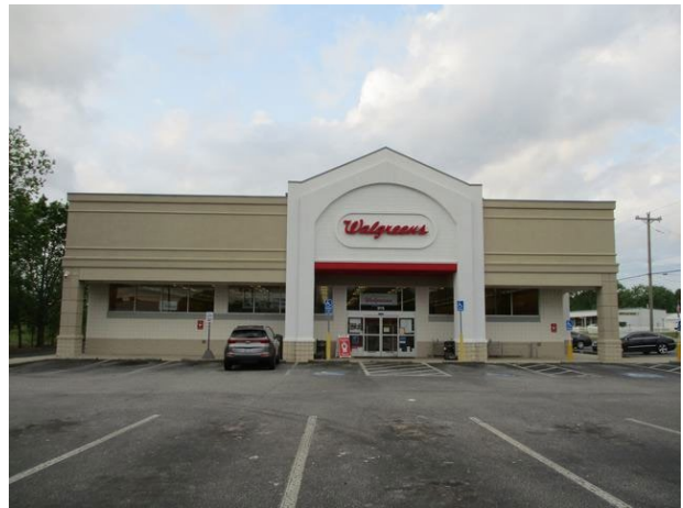
Typical commercial/retail uses in Subject's neighborhood
