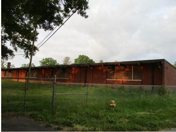
View of Subject site
